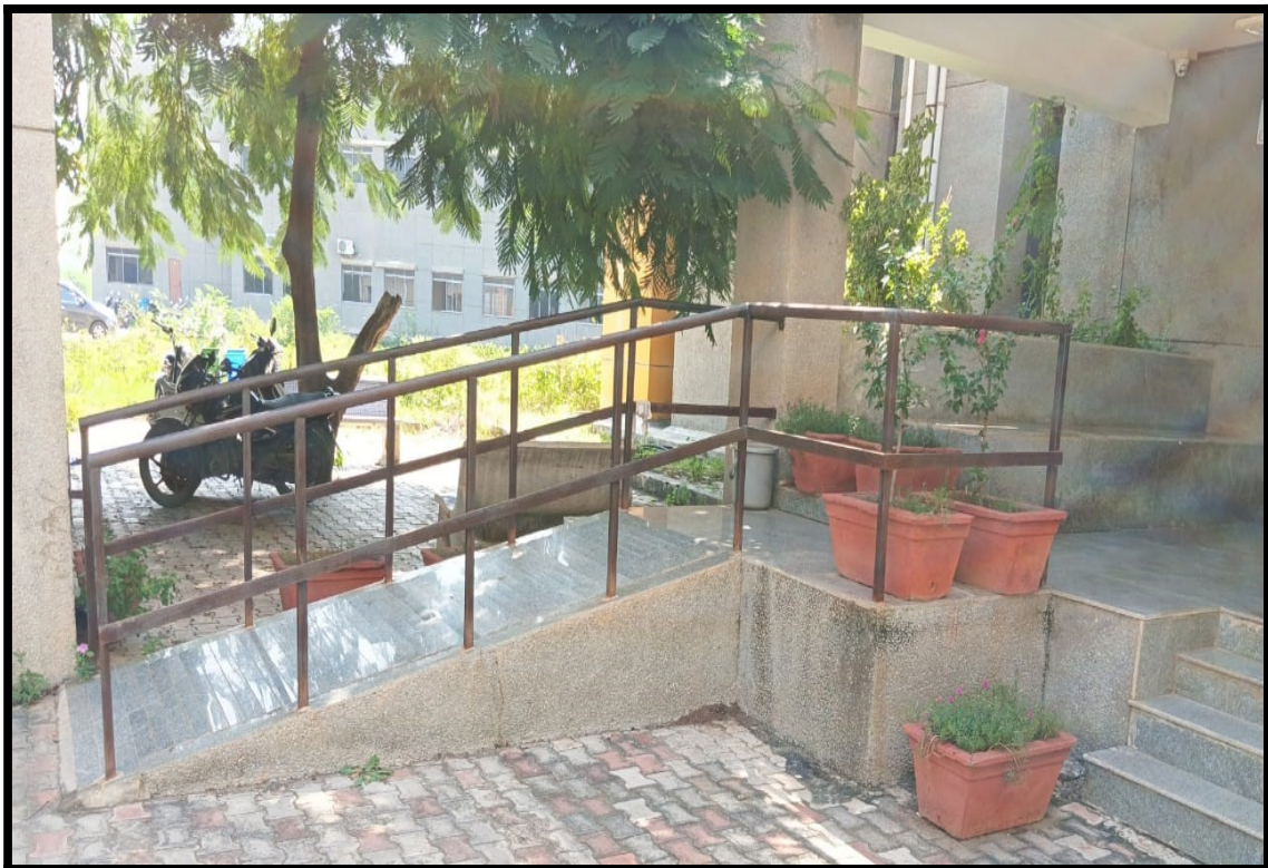
RAMPS WITH RAILINGS
